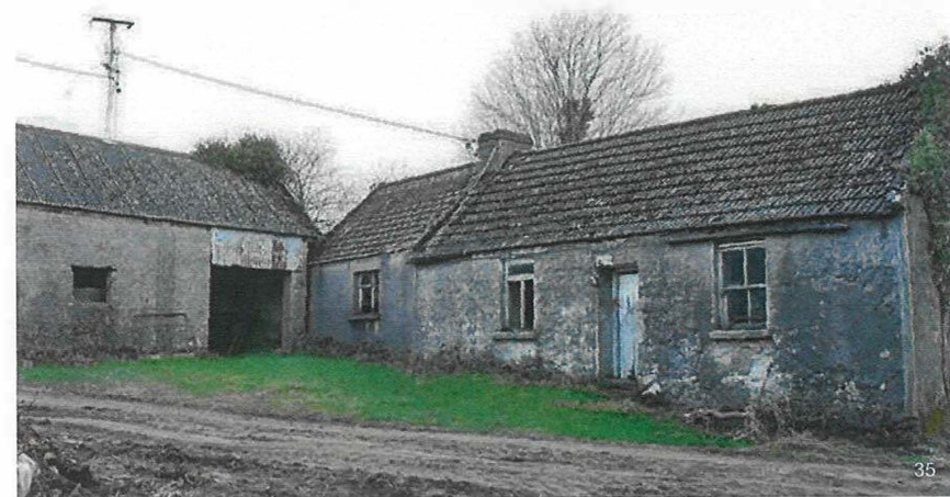
Restoration potential of cottage and outbuildings. Tinahely, County Wicklow.
